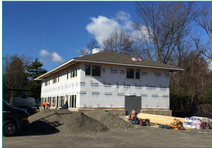
Axley Place under construction
