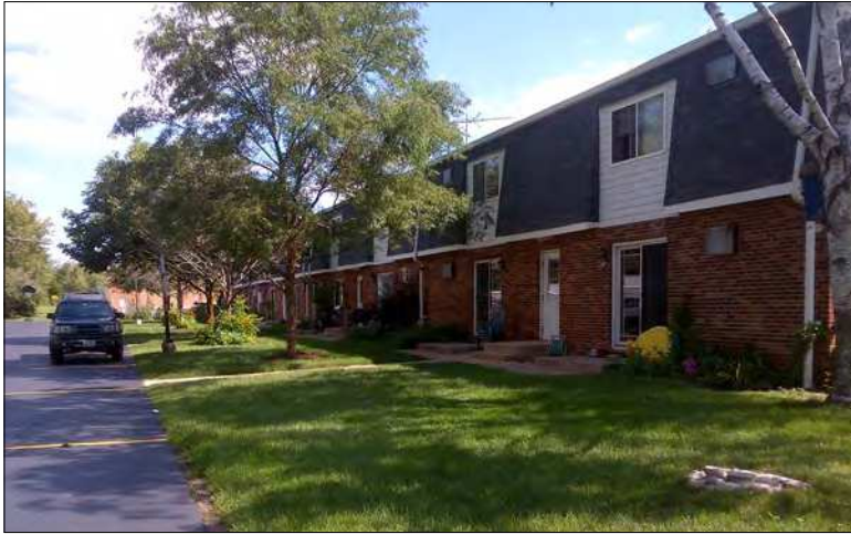
HODC acquired Towerview Apartments in McHenry.
