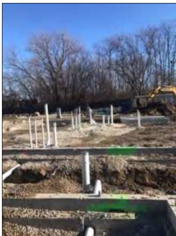
Heart’s Place under construction.
